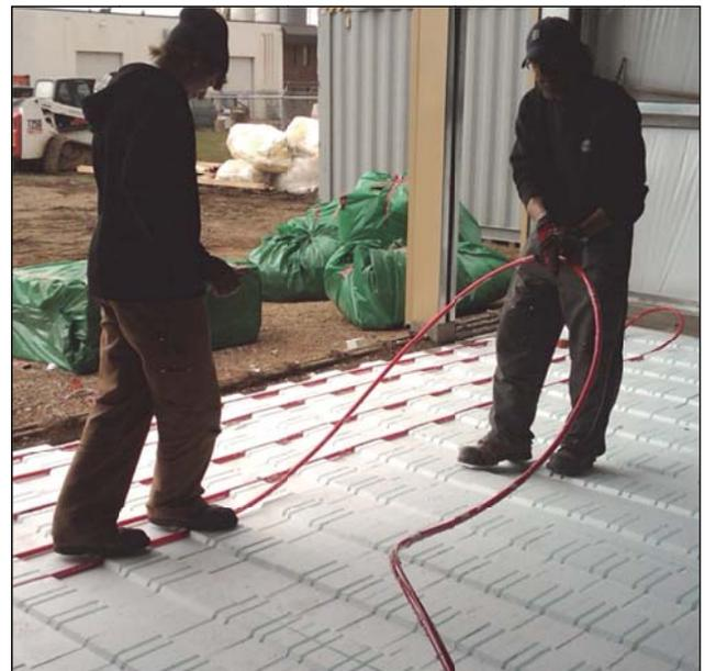
PlastiSpan HD hydronic insulation is an expanded polystyrene (EPS) insulation used as the insulation component in radiant floor heating systems. PlastiSpan HD hydronic insulation decreases heat loss to ground, allows uniform heat distribution to the floor area above and ensures the floor area will be warmed faster.
